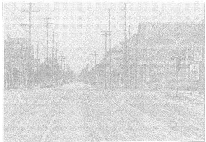
Flashing signal at Shelby street crossing of Belt railroad
